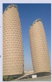
The buildings are over-clad on the south, east and west sides by a unique dynamic shading system, that opens and closes to provide self shading as the sun moves around the building. This system is predicted to reduce the solar energy entering the building by 20% and is one of a number of innovative measures to enhance environmental performance and limit energy use. The project has been designed in accordance with the US Green Building Council LEED rating system.
